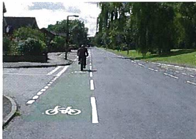
Example: Advisory cycle lane with full green colouring over side road junctions
