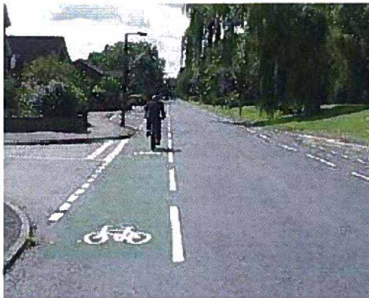
Example: 2 metre cycle lane with full green colouring over side road junctions
