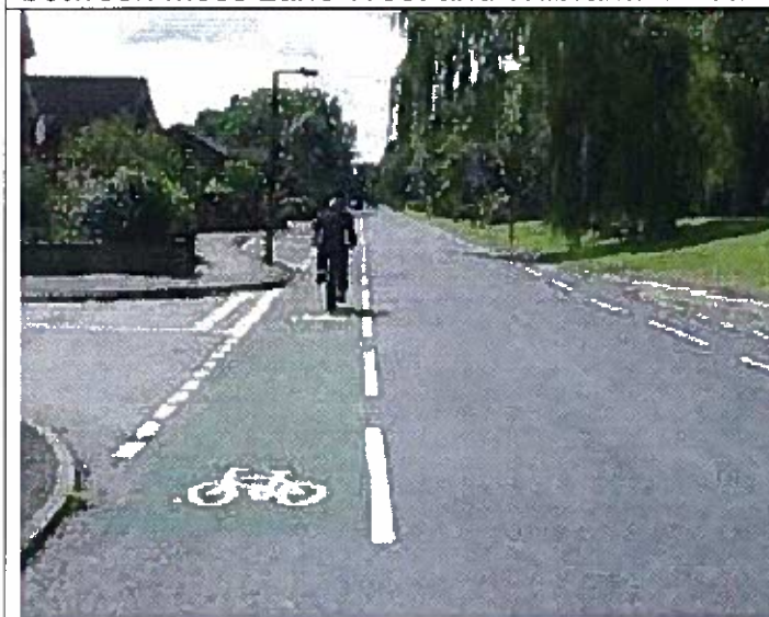
Example: Advisory cycle lane with full green colouring over side road junctions
