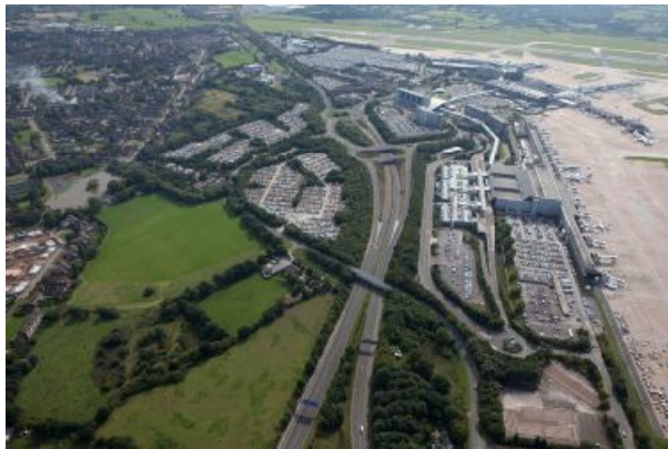
Existing Site Aerial
