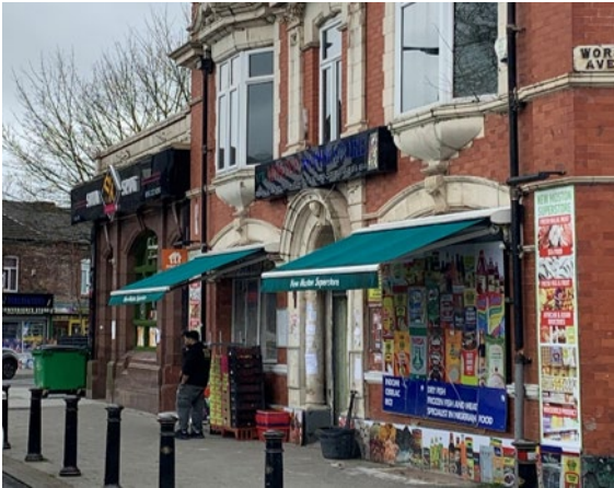
Figure 3: New Moston Superstore occupies a prominent Victorian corner building at the eastern end of the centre and serves as one of the primary convenience anchors for the local community.
