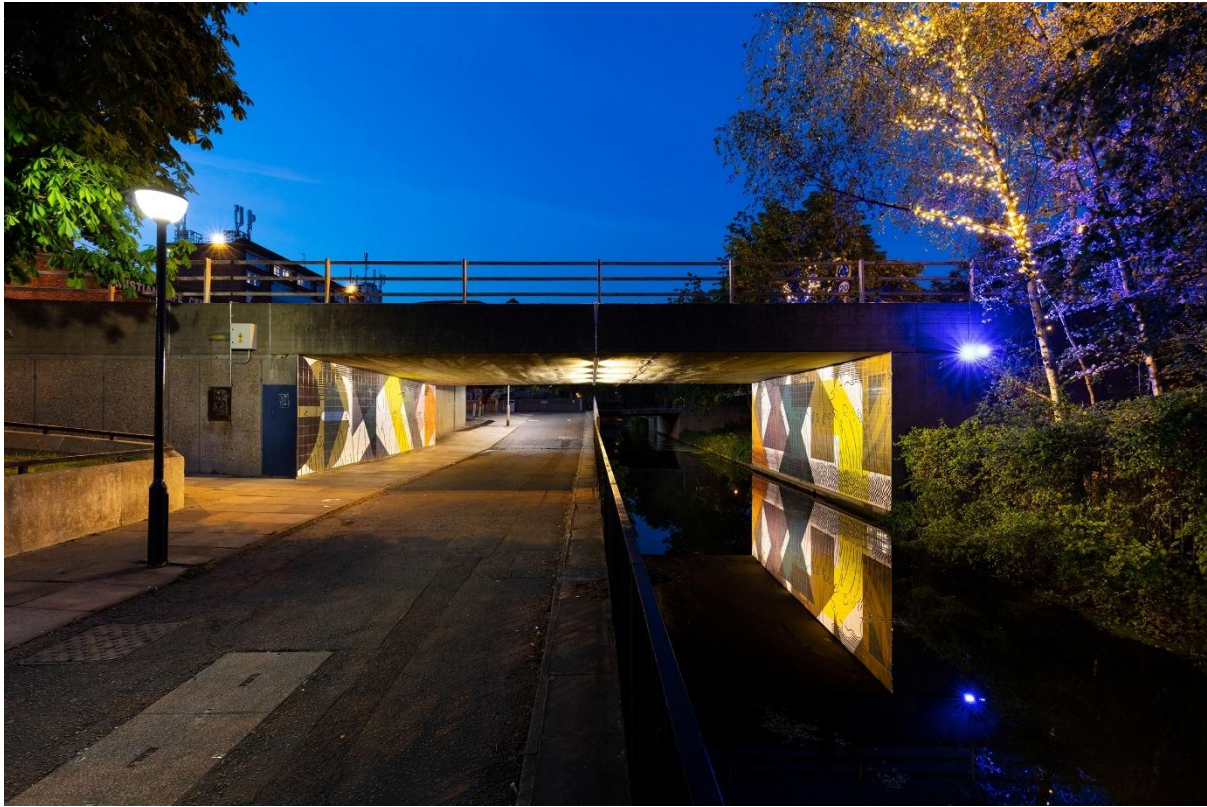
Figure 56: The Moorings - Moorings underpass Thamesmead. Tile installation by Grantchester Pottery. Lighting by Light Follows Behaviour.
