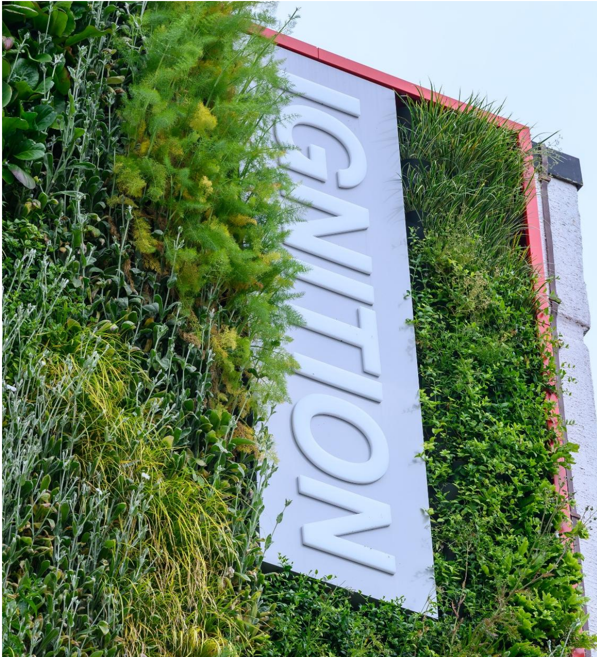
Figure 79: Cockcroft Building with green wall and nest box (© Salford University)
