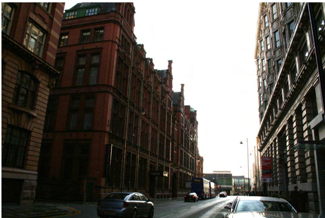
Plate 30 Whitworth Street. Early 20 th century shipping warehouses
