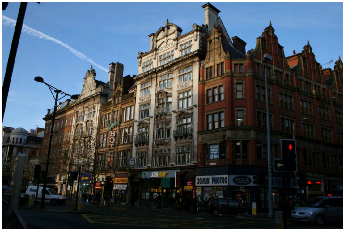
Plate 32 Piccadilly area. Late 19 th to early 20 th century commercial warehouse
