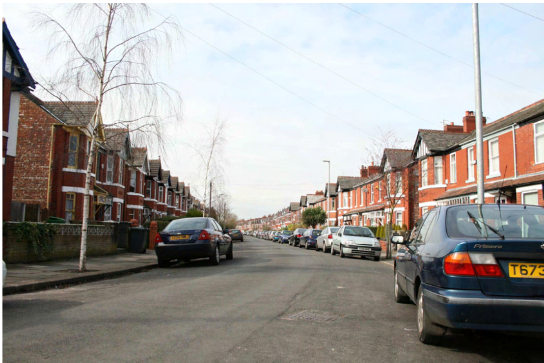
Plate 12 Nicholas Road, Chorlton-cum-Hardy. Late 19 th to early 20 th century higher status terraced houses
