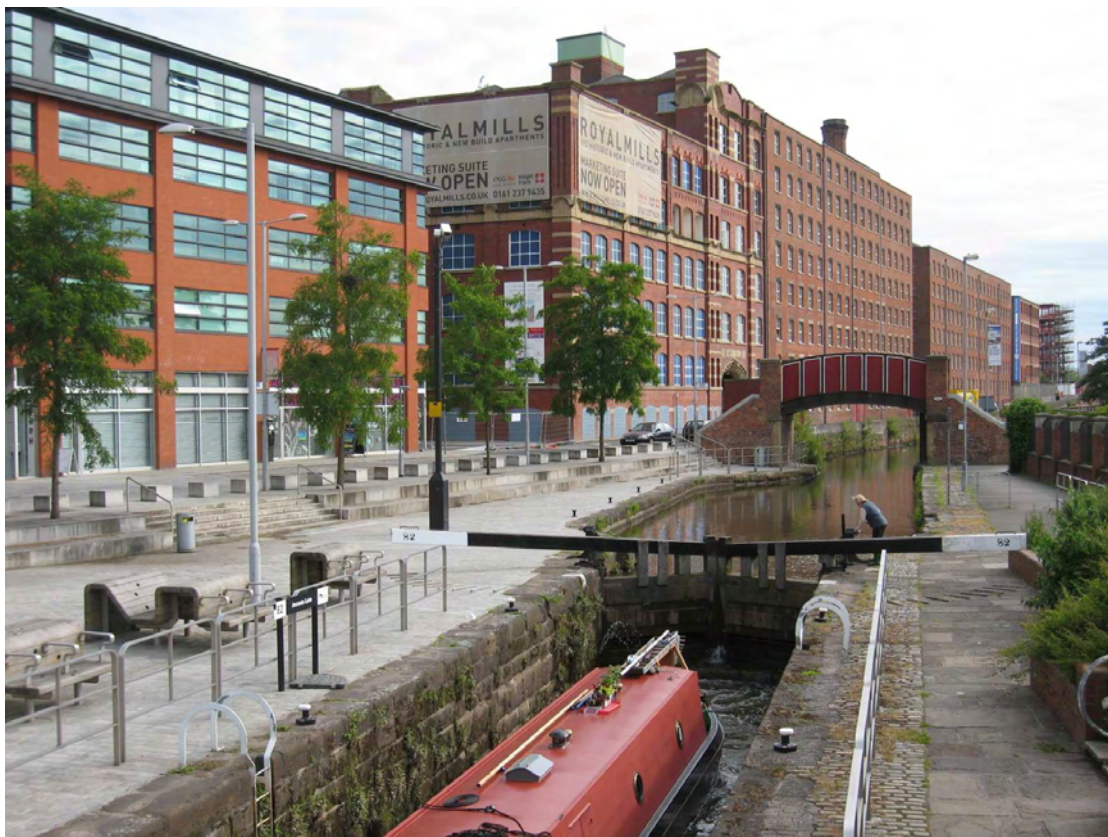
Plate 20 Ancoats mills and Rochdale Canal
