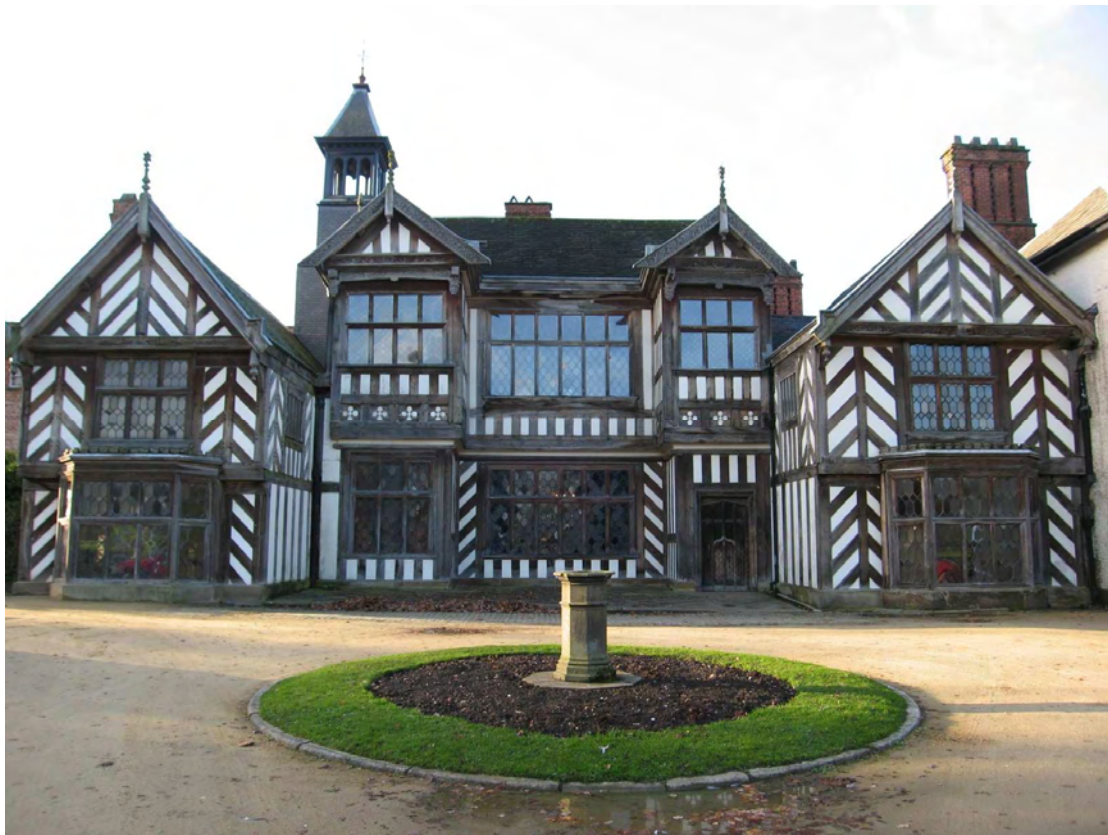
Plate 4 Wythenshawe Hall, south elevation. Post medieval double cross wing hall
