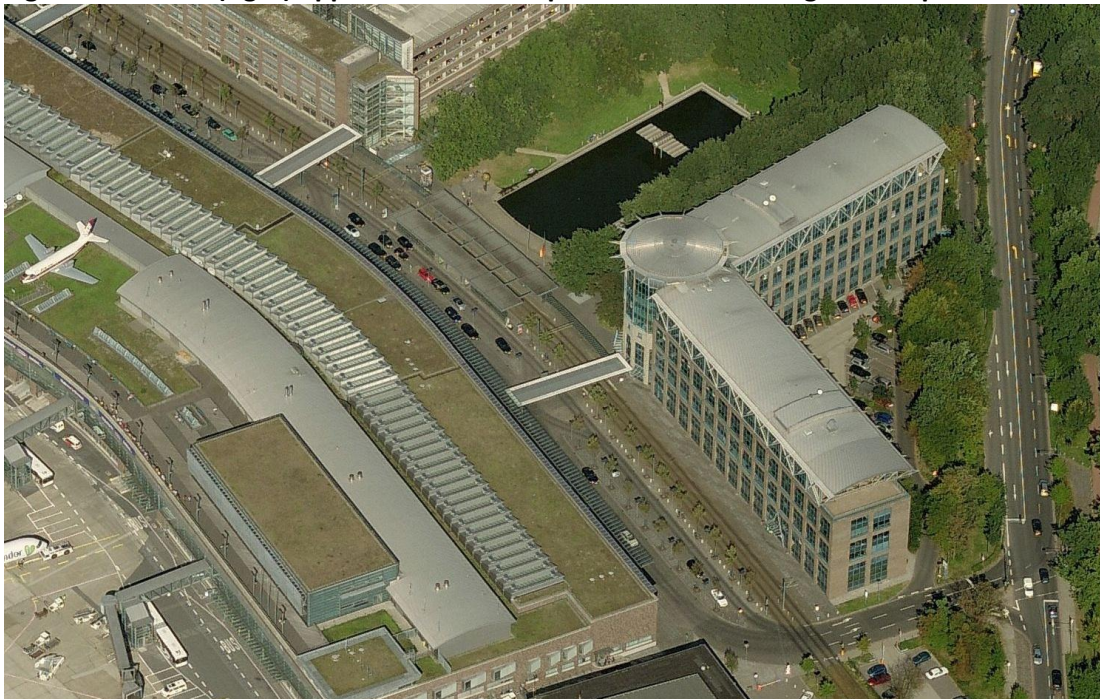
Figure A3 Offices (right) opposite Bremen airport terminal showing tramstop
