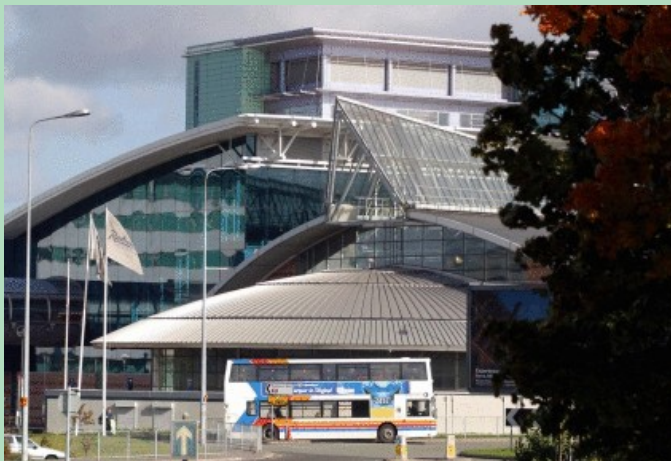
Picture 5.16 The Station
