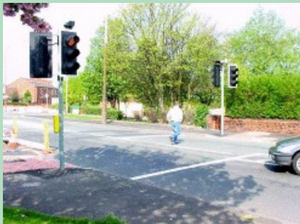
Picture 5.6 New pedestrian crossing, Tameside
