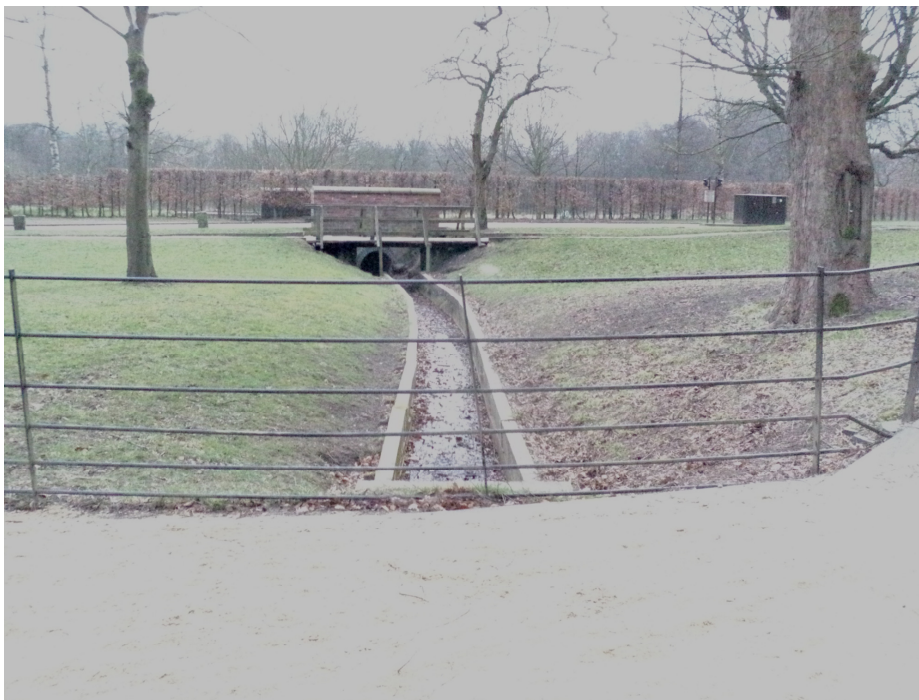
Figure 1A: Example of inlet structures for ordinary watercourses in Manchester (Good condition)
