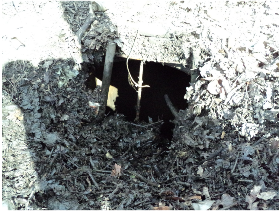
Figure 1B: Example of inlet structures for ordinary watercourses in Manchester (Bad condition)
