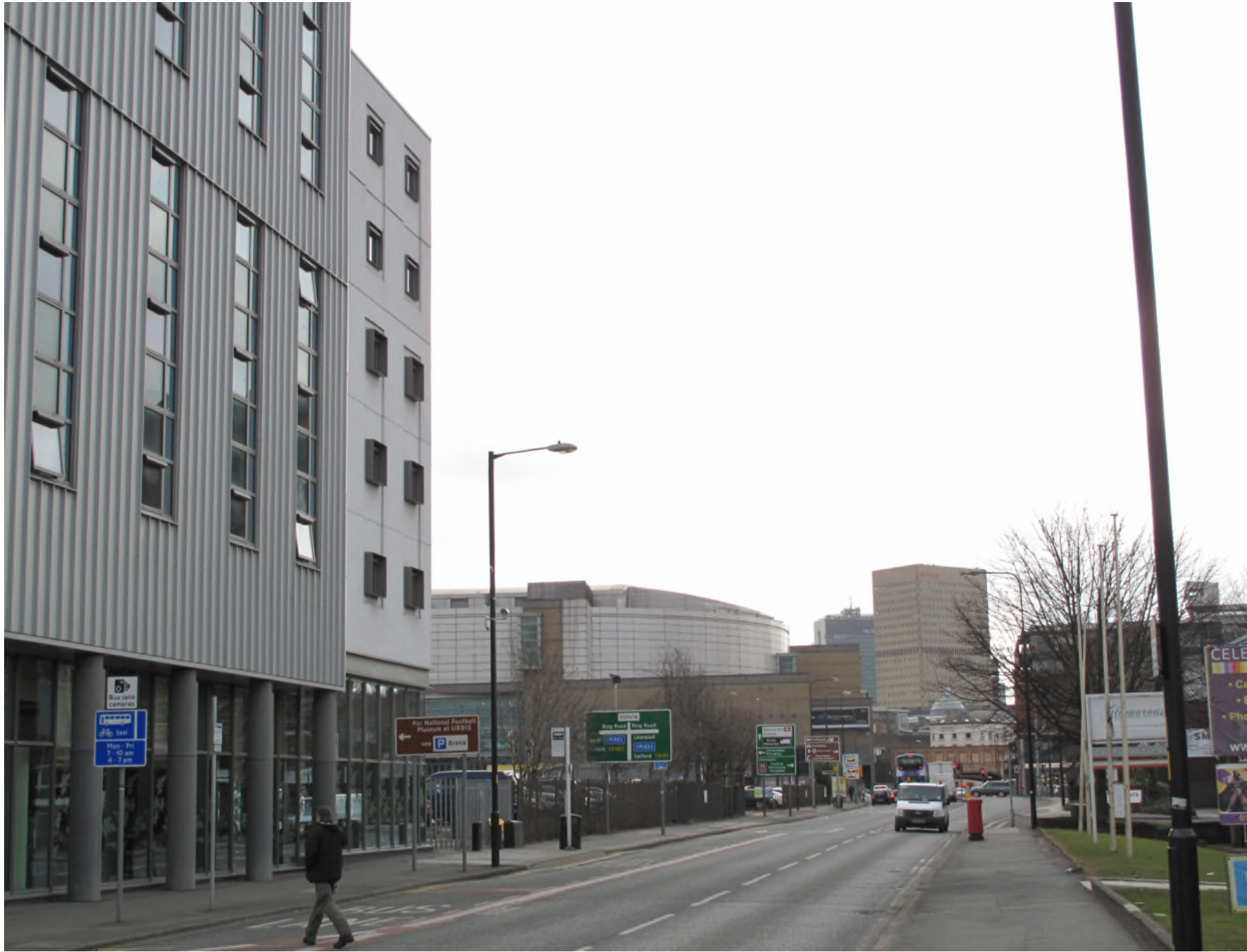
Figure 5.9 - View South from Great Ducie Street
