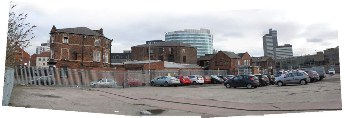
View 2 – Dutton Street from upper car park
