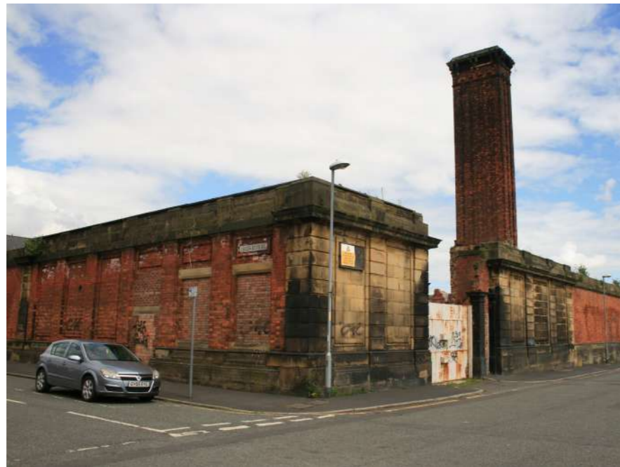
Highway lighting column
