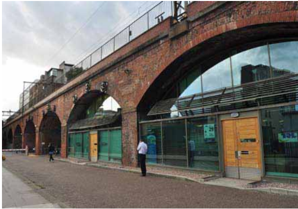
Reuse of railway arches - Altrincham Street
