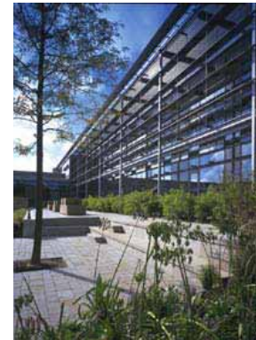
Wessex Water (Bennetts Associates, Buro Happold and Davis Langdon)
