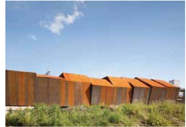
Piccadilly Place substation
