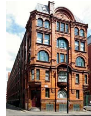
—Langley Buildings, Dale Street, Grade II Listed
