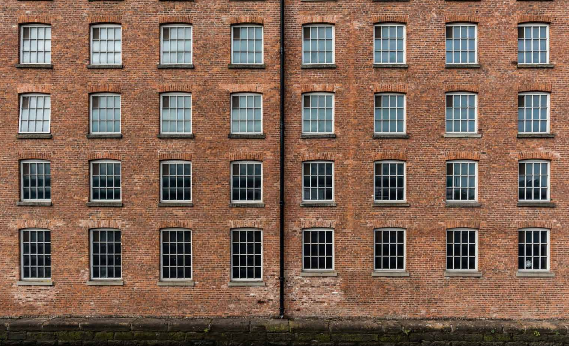
Brownsfield Mill, part of the rich context of Ancoats which is to be respected and extended.
