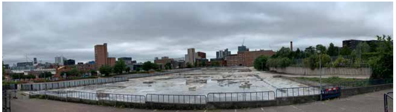
The site perimeter contains a significant level difference of over 5m
