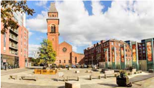
Ancoats - Cutting Room Square
