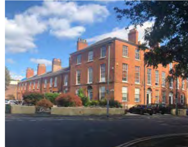
2-6. 21, 23, 25 and 27 MANOR STREET, 27 and 29 ARDWICK GREEN NORTH GRADE II (List Nos. 1219791, 1283018, 1219817, 1207536, 1283046)
