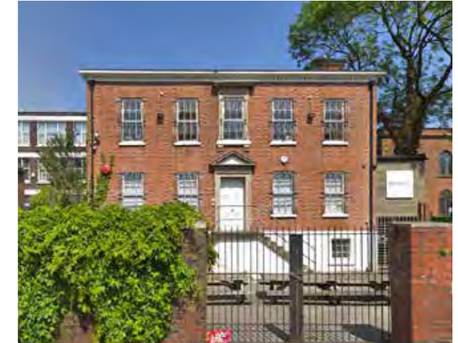
6. MILFORD HOUSE, 29, ARDWICK GREEN NORTH, GRADE II (List No. 1283046)
