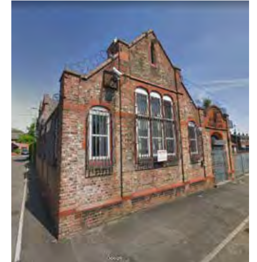
4. The Old School House, Thirsk Street
