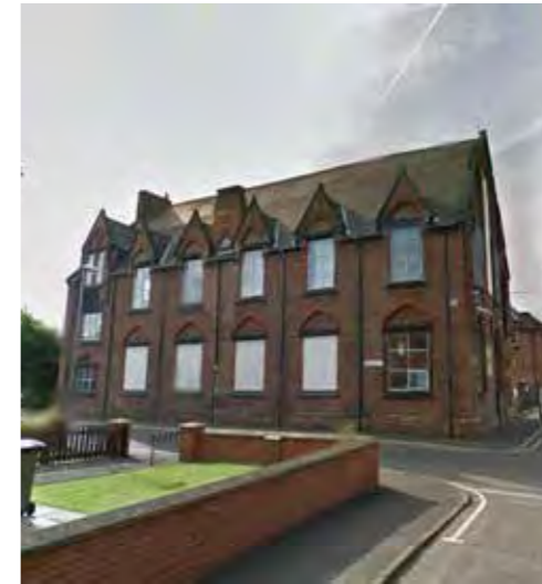
3. The Old School House, Thirsk Street
