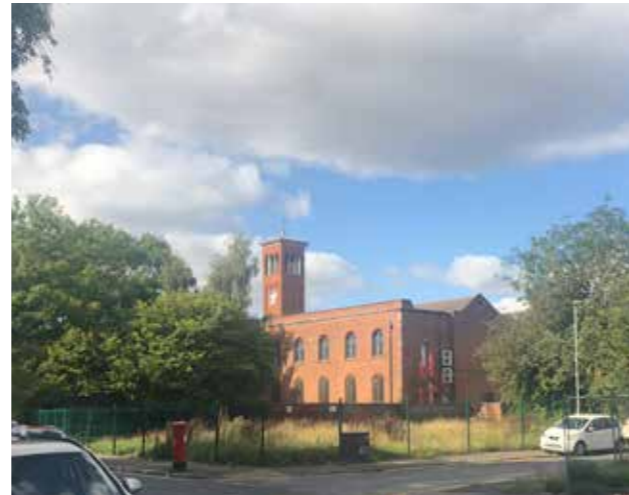
8. FORMER CHURCH OF ST THOMAS, ARDWICK GREEN NORTH, GRADE II (List No. 1197828)
