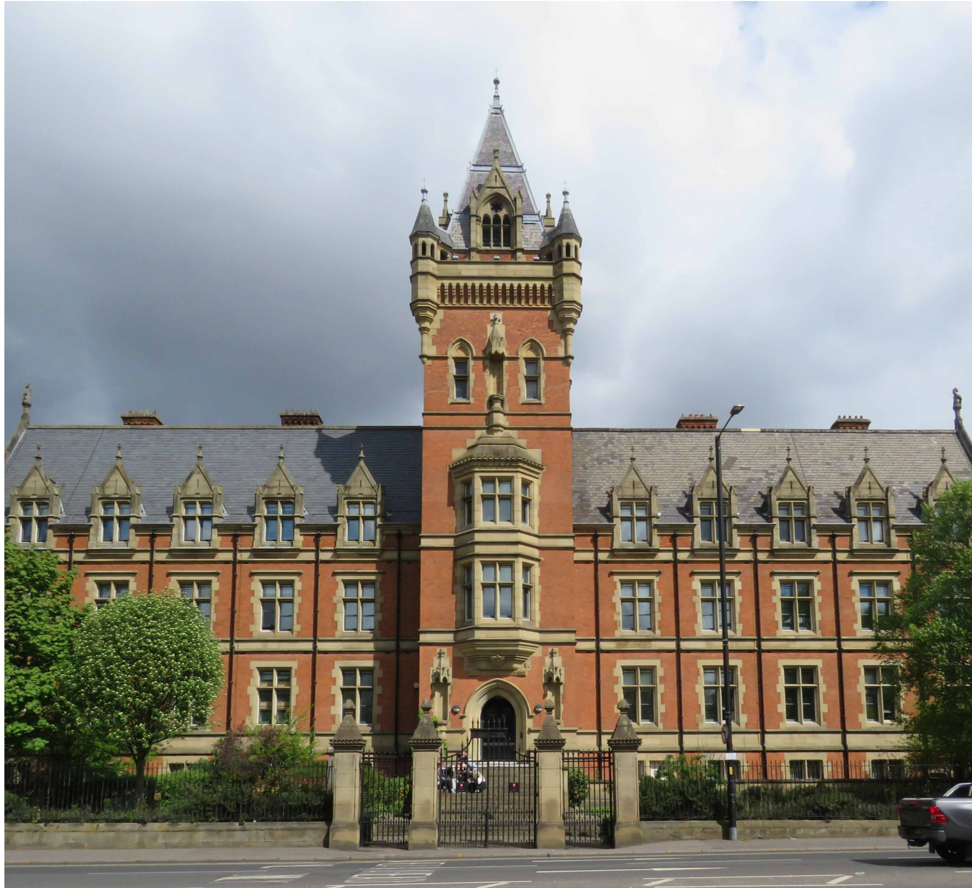
Nicholl's Building. The Manchester College
