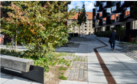
Filter drains integrated into spaces
