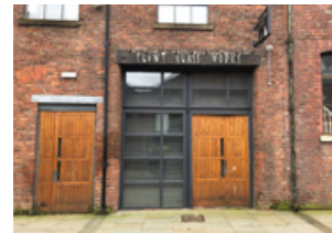
Red brick facade with stone sills and timber
