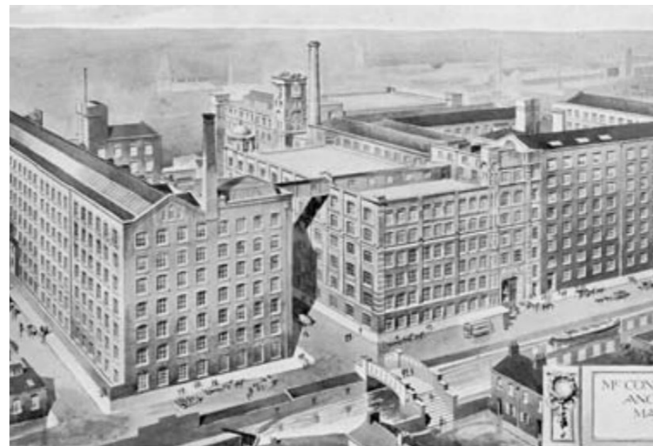
Long Mill and Old Mill defining the frontage of Rochdale canal in 1913 Source: 'Ancoats. Cradle of industrialisation.' English Heritage
