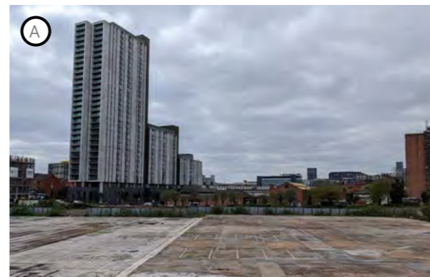
View across the site towards the Great Ancoats Street, Oxygen tower on the left.
