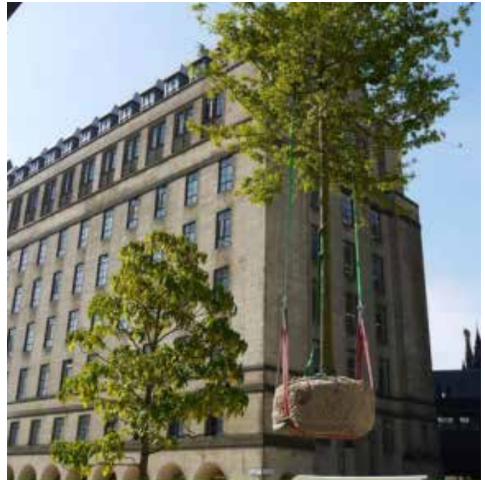
Photograph showing trees being craned into position in St Peter's Square, 2016 – Source; Manchester City Council.
