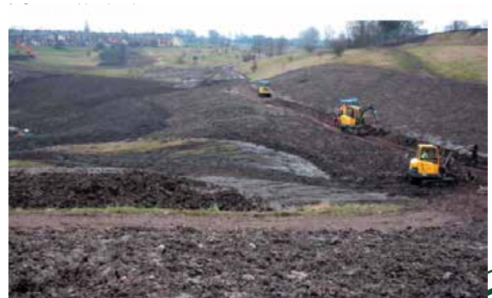
Photograph of site preparation works on Moston Vale in 2006 – Source; Newlands
