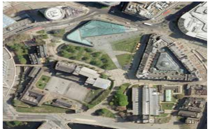
Aerial view showing Cathedral Gardens in 2021 – Source; © Getmapping Plc and Bluesky International Limited 2021
