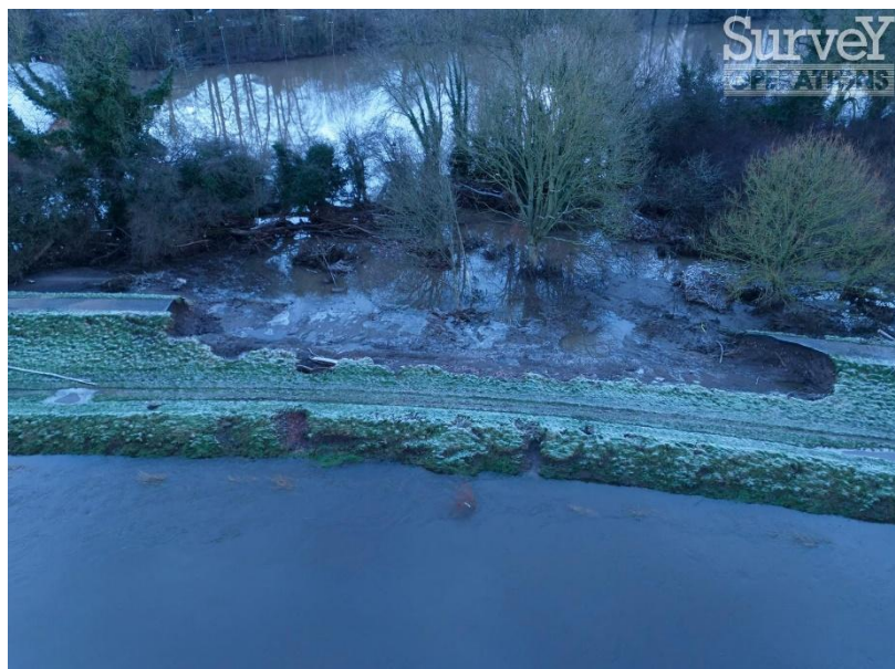
Figure 7. Drone photograph of the River Mersey embankment breach at Ford Lane, taken 03/01/2025.
