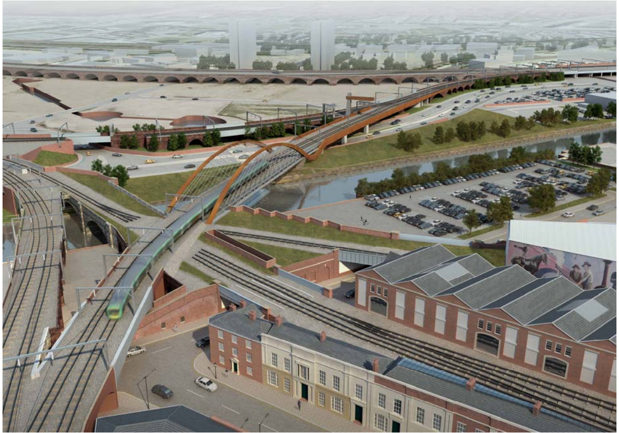
Figure 7: Bowstring bridge option looking towards Salford from Liverpool Road, Manchester
